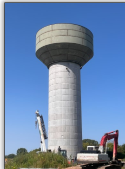
Northeast Water Supply Tower
