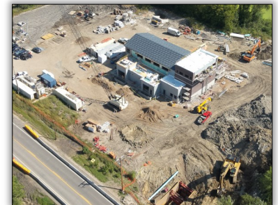
Northeast Water Treatment Plant
